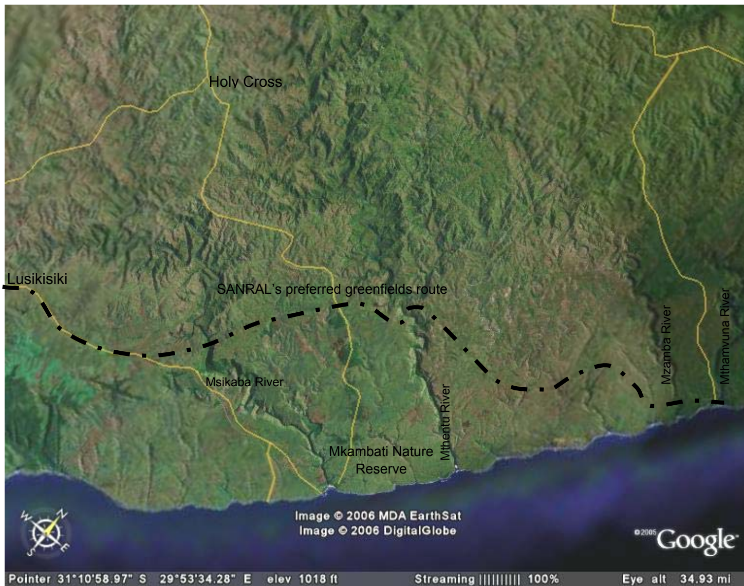
Figure 6.1: Satellite image of topography in the study area between Lusikisiki and the Mthamvuna River, with SANRAL's preferred greenfields route through this section
