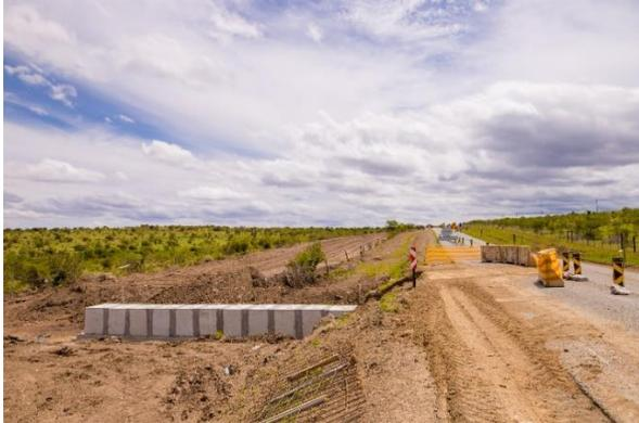
**Box culverts are being installed to accommodate the storm water under the existing road. Temporary pipes are placed under the deviation to accommodate rainwater flowing through the existing culvert.**
