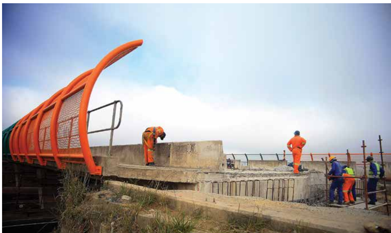
Work in progress on the Thembaletu Bridge in George, which was completed in 2024
