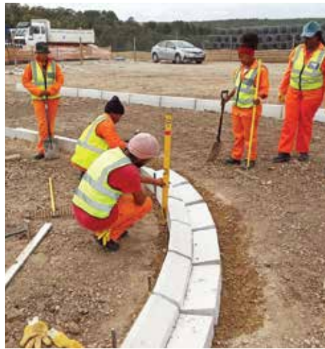
Laying and setting out kerbs and channels on the Kraaibosch to Touwriver project
