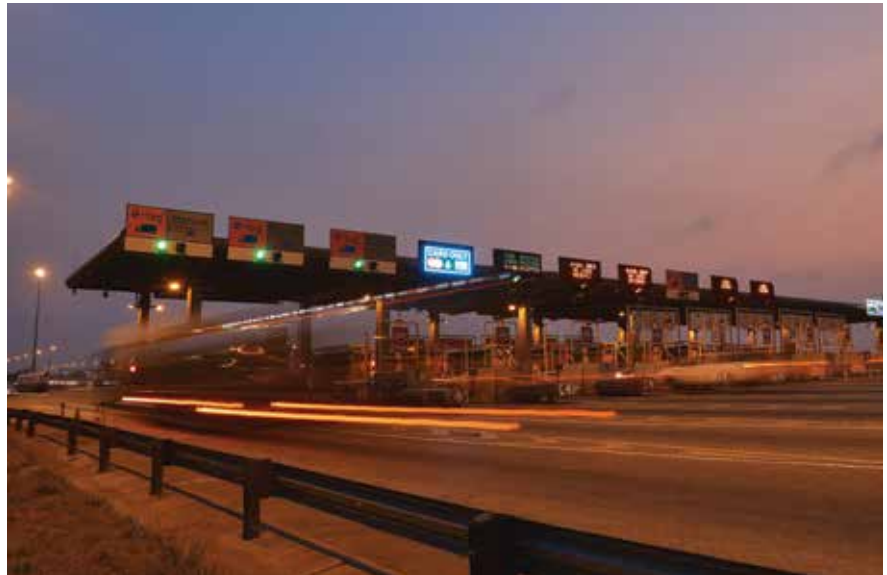
Toll plaza on the Bakwena N1N4 toll route
