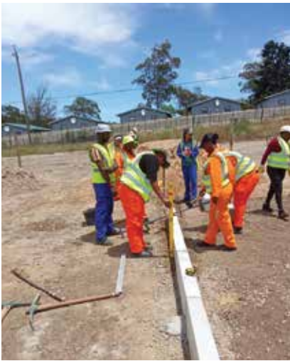
Laying and setting out kerbs and channels on the Kraaibosch to Touwriver project
