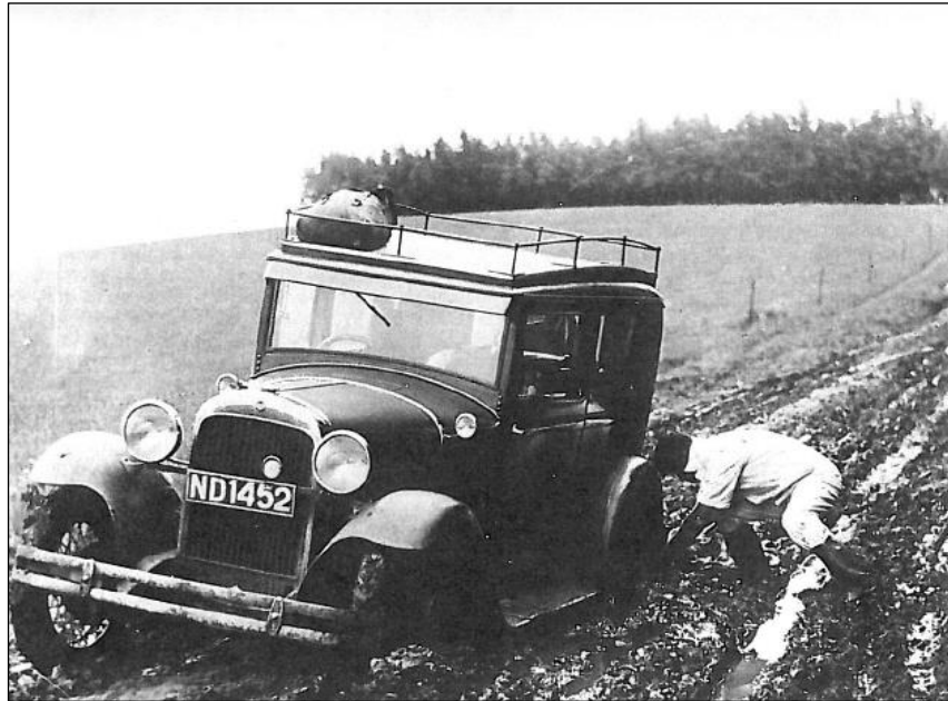
Figure 5. Impassable Unsurfaced Roads Due to Wet Conditions, Early 20 th Century
