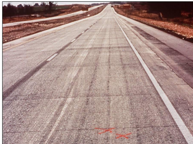
Figure 60. Vibrator Trails
