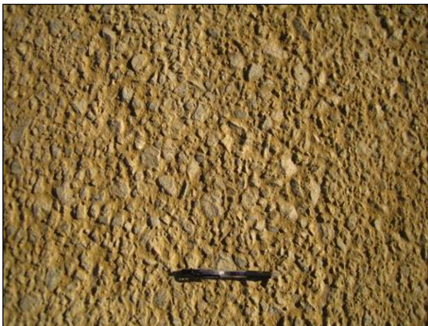
Figure 81. Well-knitted Crushed Stone Surface
