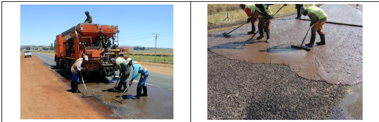
Figure 94. Slurry Placed By Hand
