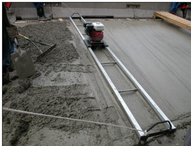
Figure 56. Surcharge in Front of Beam
