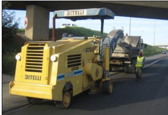
Figure 32. Small Milling Machine
