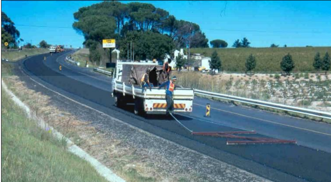
Figure 93. Z-Type Drag Broom
