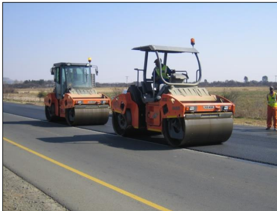
Figure 62. Double Drum Rollers
