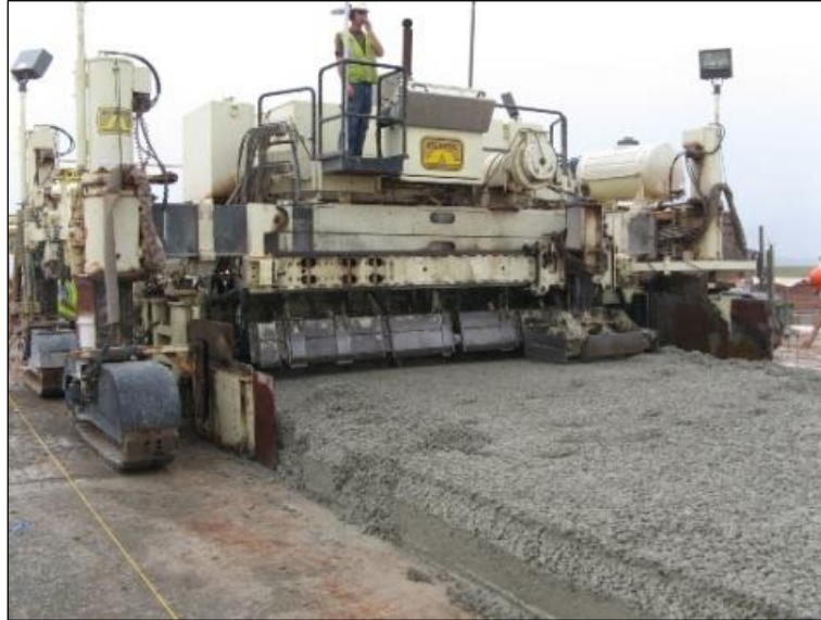
Figure 53. Slipform Paver
