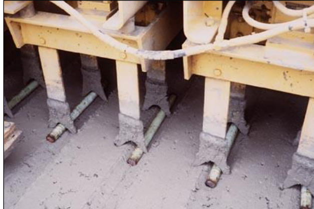
Figure 55. Dowel Bar Inserters
