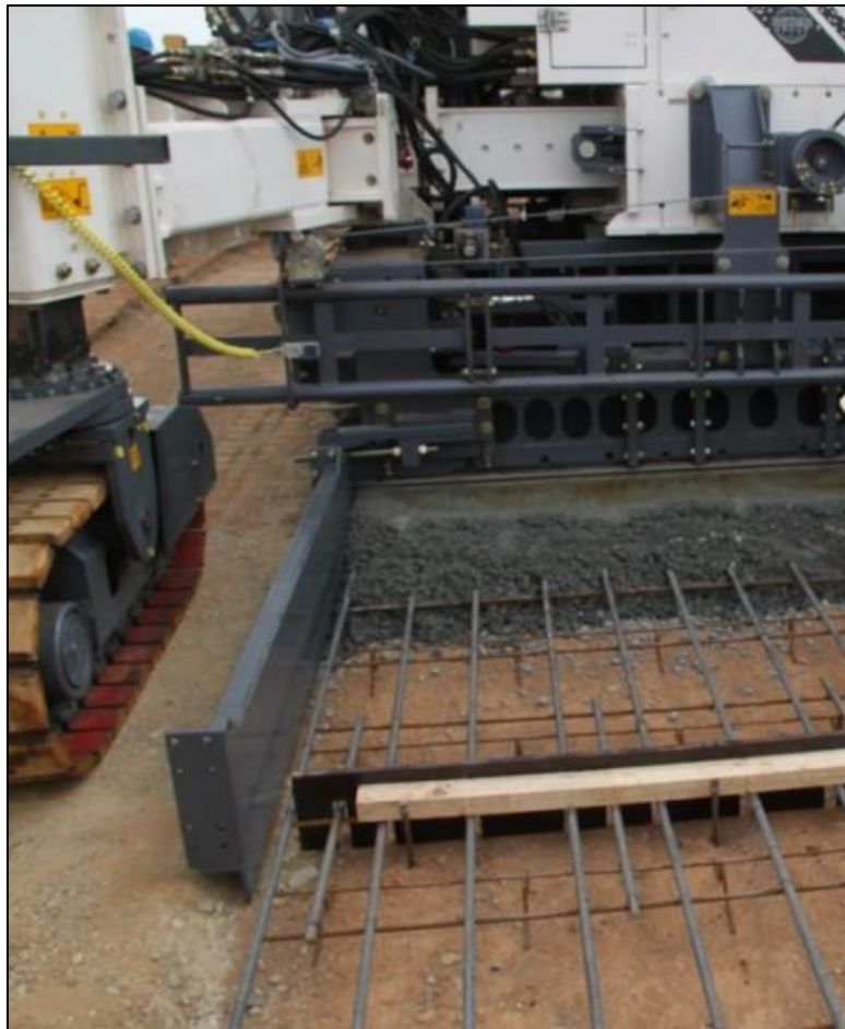
Figure 51. Concrete Placing Equipment
