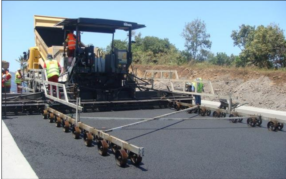
Figure 97. Levelling Beam for Level Control
