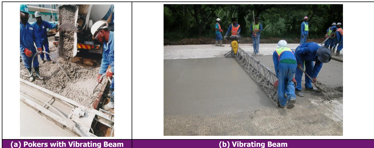
Figure 54. Vibrators
