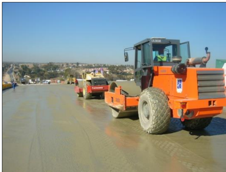
Figure 79. Compacting Crushed Stone
