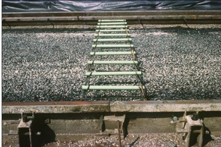
Figure 103. Installation of Dowel Bars
