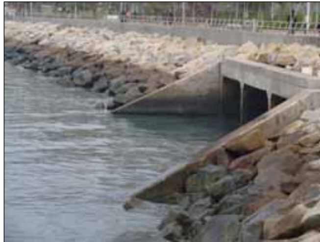
Figure 70. Removal of Stormwater by a Large Culvert
