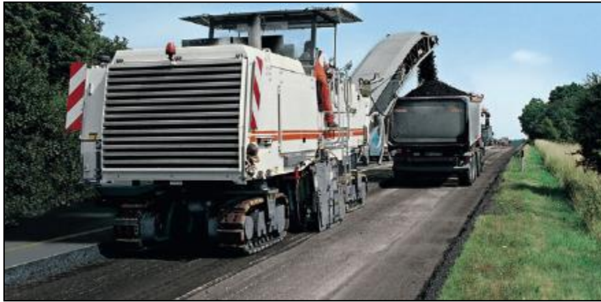
Figure 31. Example of Milling Machine
