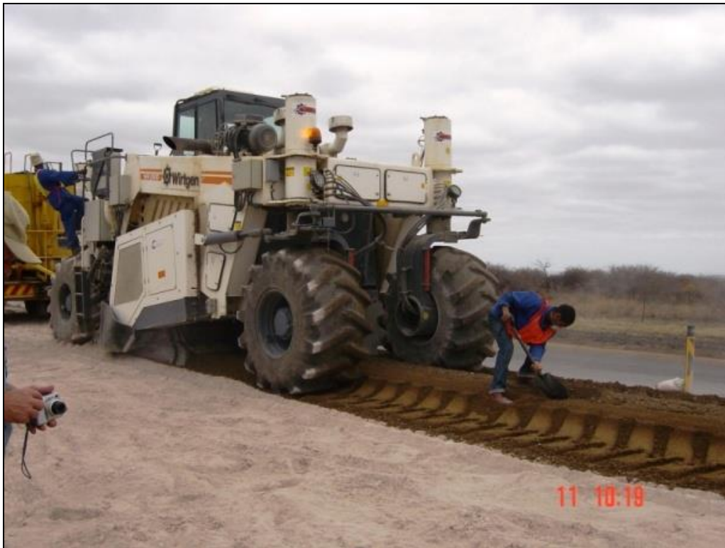
Figure 43. Example Tyre Mounted Recycler Showing Recycling Wheel Paths
