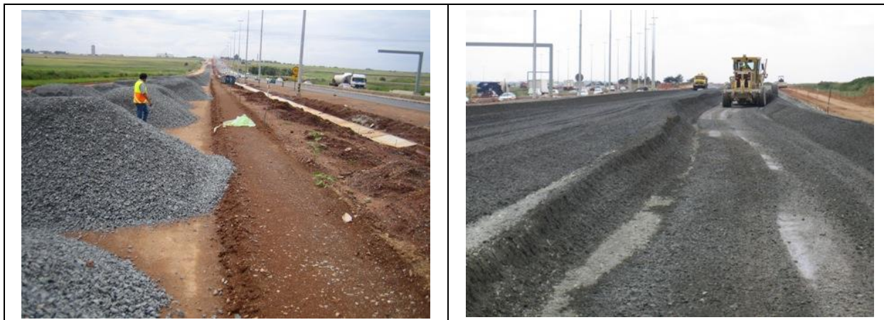
Figure 75. Dumping and Spreading of Crushed Stone
