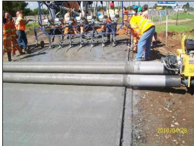
Figure 102. Strike-off Beam
