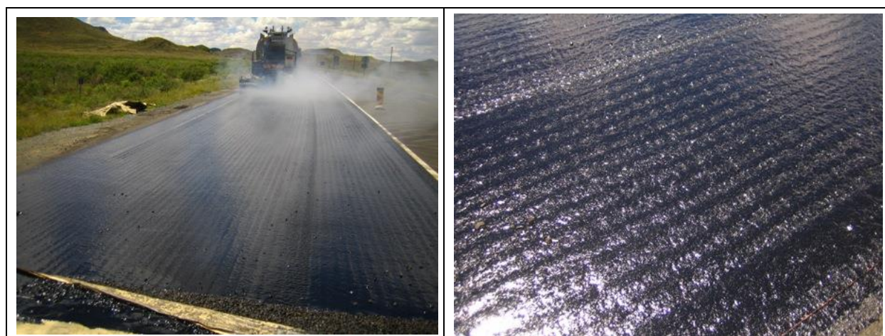
Figure 28. Streaky Sprays (Tram Lining)
