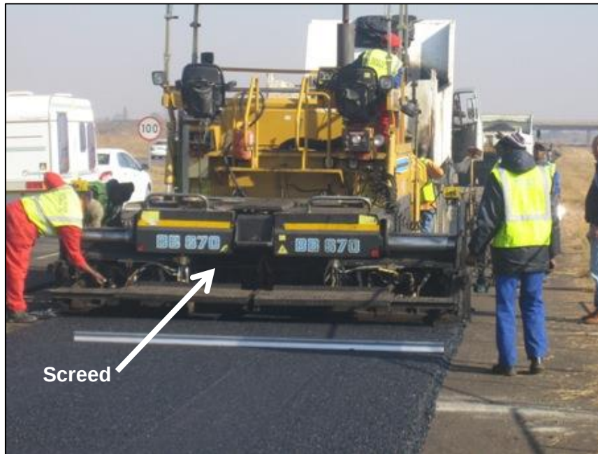
Figure 50. Screed on Asphalt Paver
