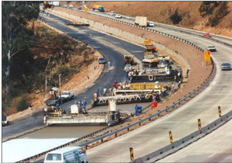
Figure 52. Fixed Form Paver
