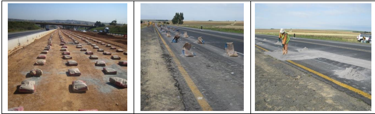
Figure 73. Bag Placement and Spreading
