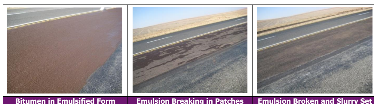
Figure 96. Slurry Setting as Emulsion Breaks
