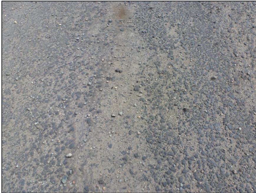
Figure 80. Segregated Material
