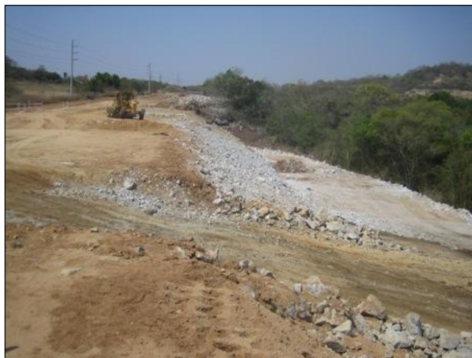
Figure 69. Rock Embankment
