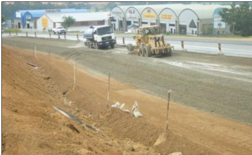
Figure 78. Mixing Crushed Stone
