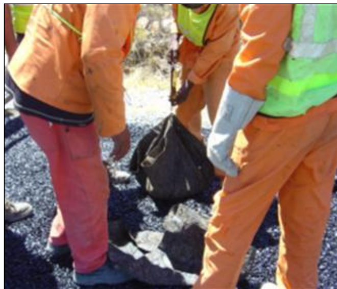
Figure 92. Measurement of Aggregate Spread Rate
