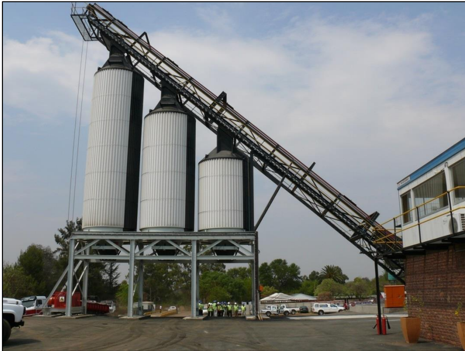
Figure 21. Hot Mix Storage Bins
