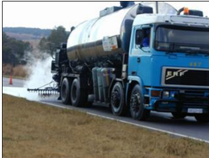
Figure 23. Binder Distributor
