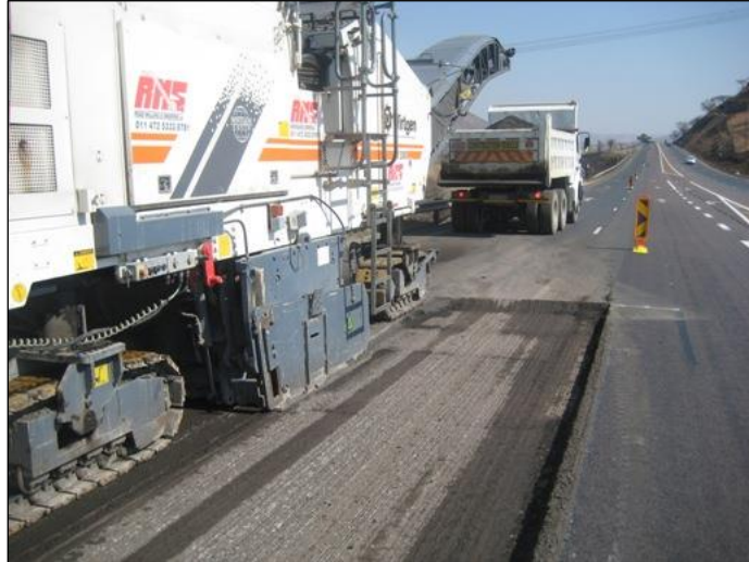
Figure 33. Large Milling Machine
