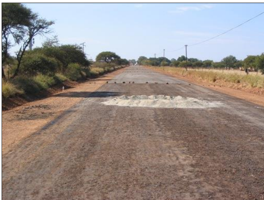
Figure 7. Carbonated Surface
