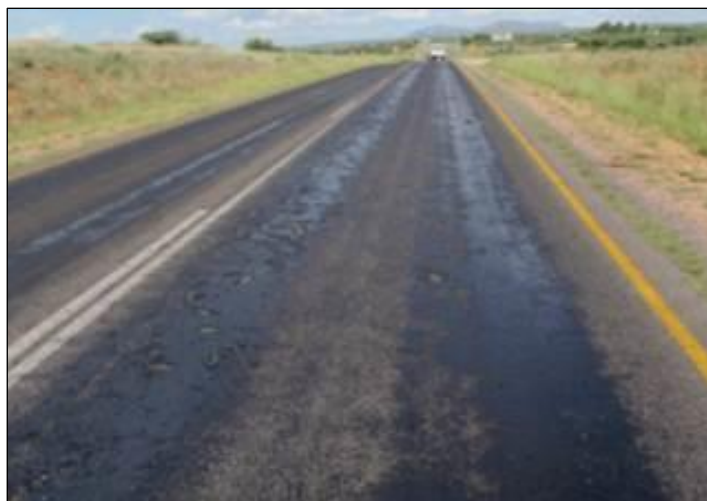
Figure 21. Bleeding Seal
