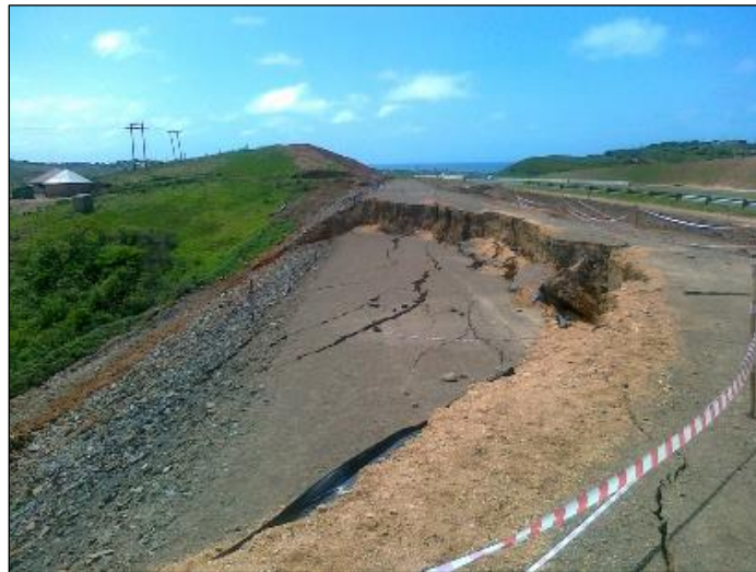
Figure 3. Embankment Failure
