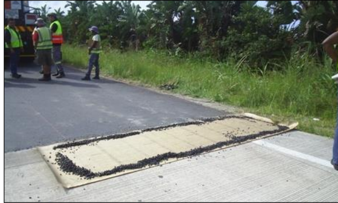
Figure 9. String Line and Reinforced Paper Strip
