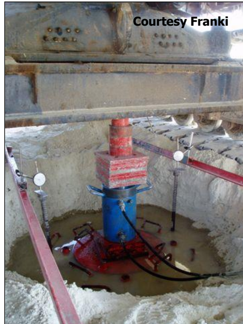
Figure 20. Plate Bearing Test
