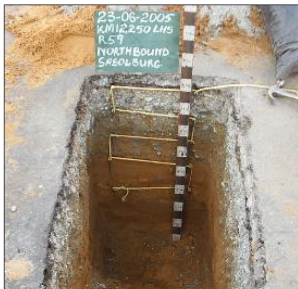
Figure 42. Example Test Pit
