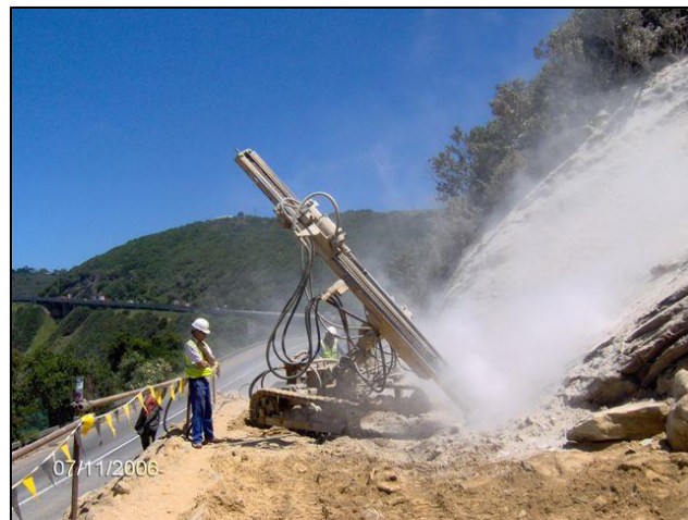
Figure 6. Percussion Drilling
