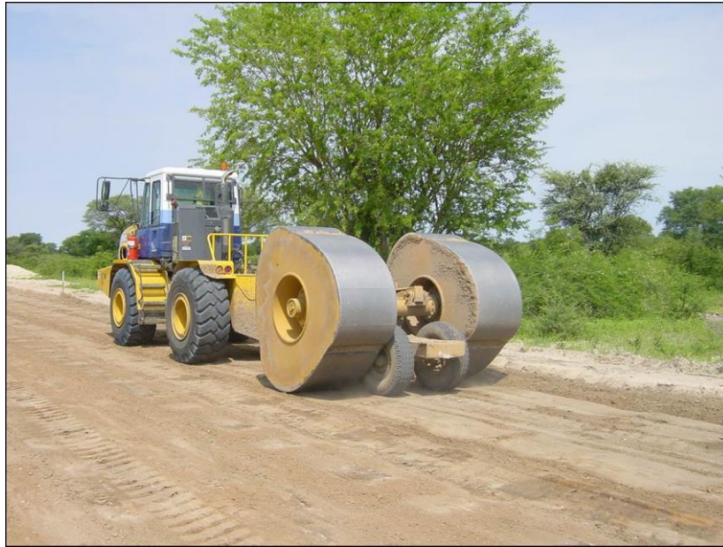
Figure 21. Impact Roller
