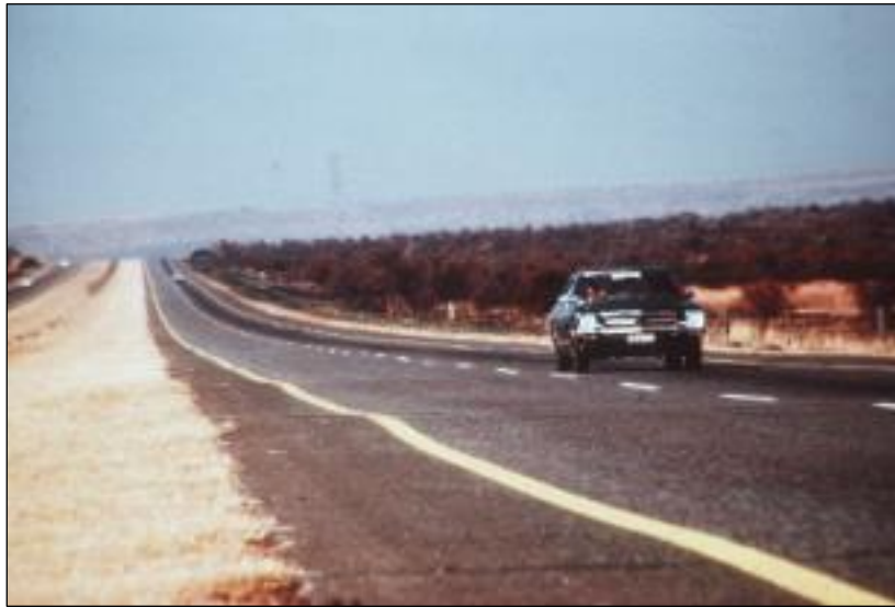
Figure 16. Unevenness and Culvert Lifting due to Expansive Clays
