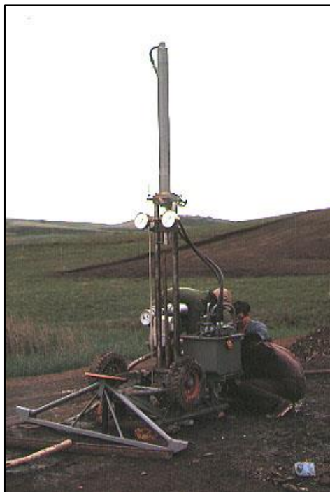
Figure 7. Cone Penetration Test
