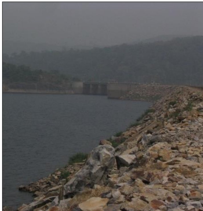
Figure 14. Large Size Blocks Used on Dam Wall
