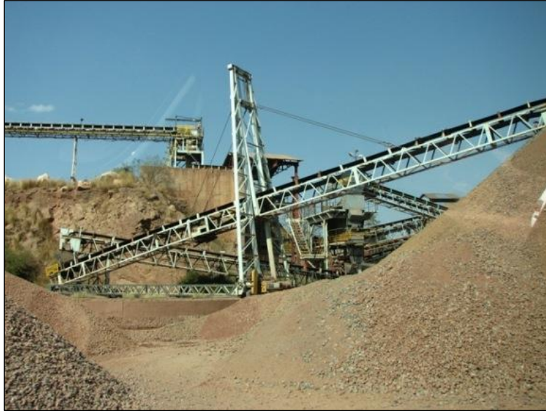
Figure 15. Mix of Rock Sizes from Crushing Operation
