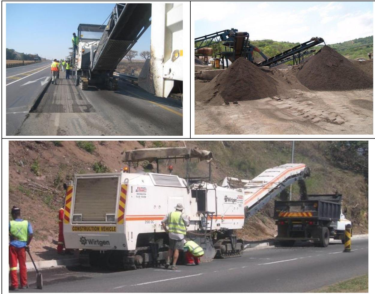
Figure 21. Reclaiming Asphalt
