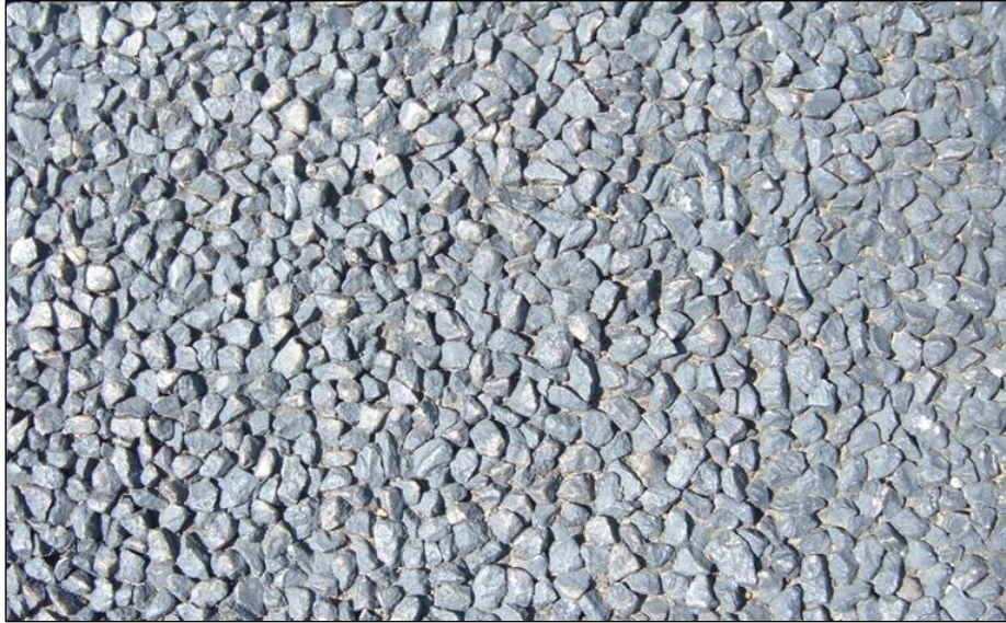
Figure 23. Steel Slag as a Single Seal
