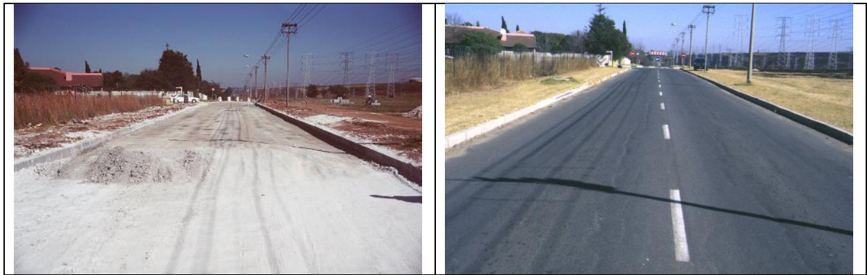
Figure 27. Example of South African Road Built with Phosphogypsum
